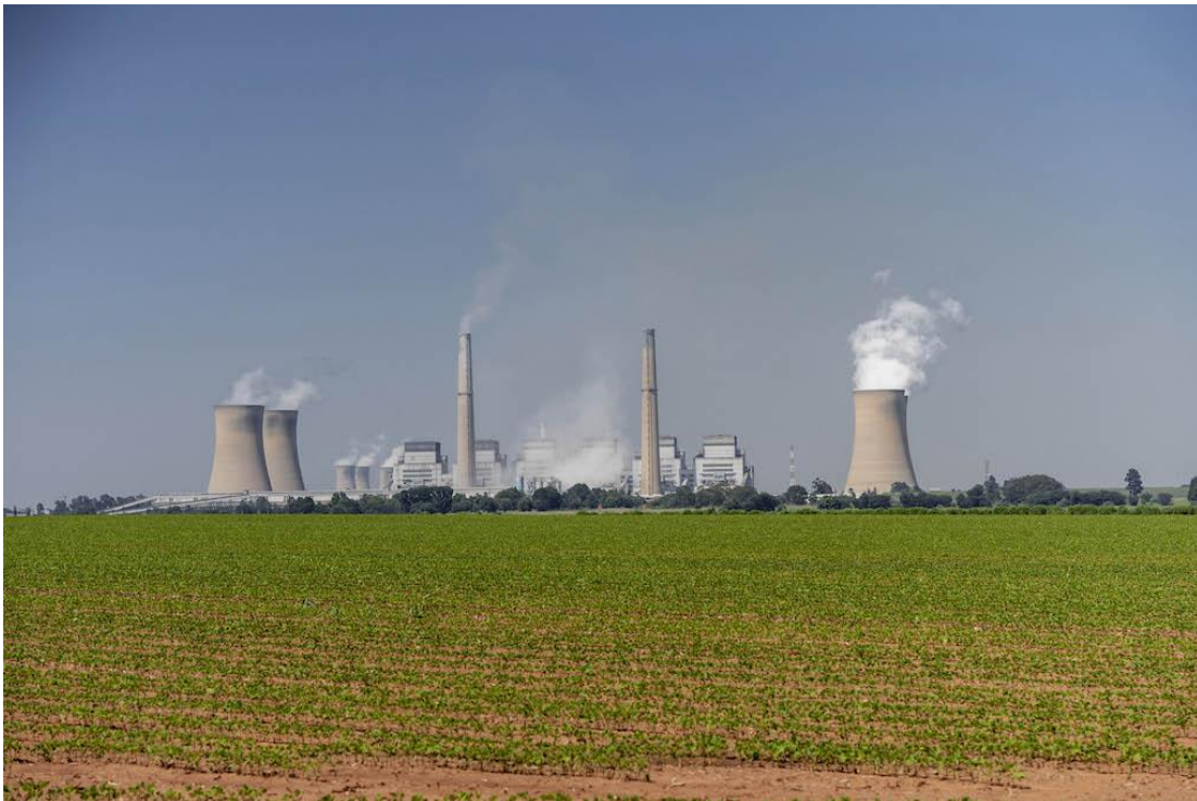
The JET Investment Plan has allocated R1.6-billion for pilot skills-development centres in several provinces, including Mpumalanga. Pictured here is Kriel power station in Mpumalanga. Photo: Ihsaan Haffjee
