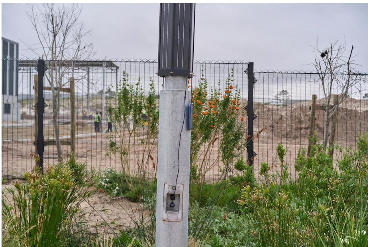
The streetlights in Zone 1 are solar powered and many of them have mobile phone charging points as well. Photo: Barry Christianson
