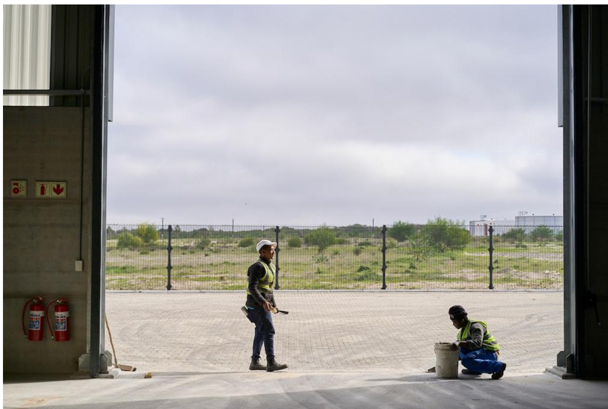
Local manufacturers, such as Ener-G-Africa, see a bright future in the localisation of renewables. Here, two artisans seal the entrance to a building under construction in Zone 1 of the Atlantis SEZ. Photo: Barry Christianson
