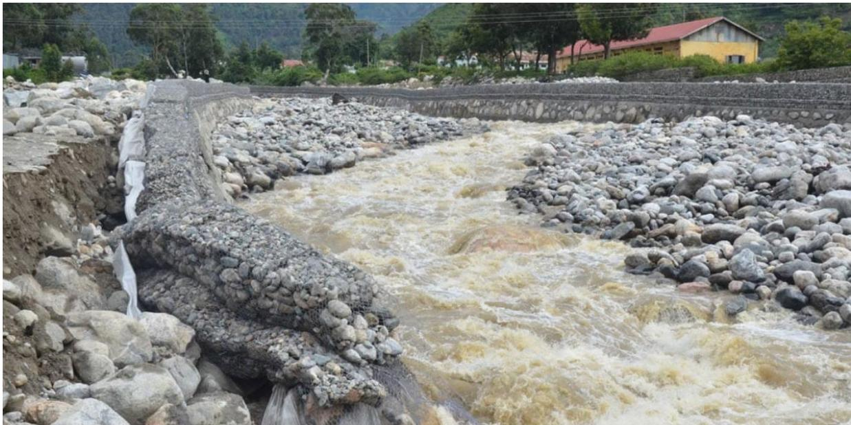
*Floods in Kasese destroyed gabions that were constructed by Ambitious Construction Company Limited on River Nyamwamba in Kasese Municipality. PHOTO/JOEL KAGUTA*
