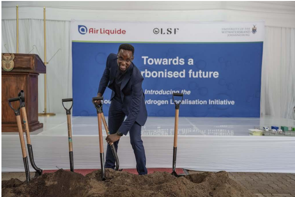
Professor Rodney Genga, assistant dean of strategic projects at the Wits Faculty of Engineering and the Built Environment, said the biggest barriers to hydrogen development are technical expertise and financing. Photo: Ihsaan Haffejee
