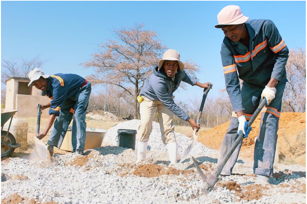
Trained mason Atamelang Matale (centre) and two colleagues mixing concrete needed to build a 'mammoth' biogas digester. Photo: Sharon Tshipa
