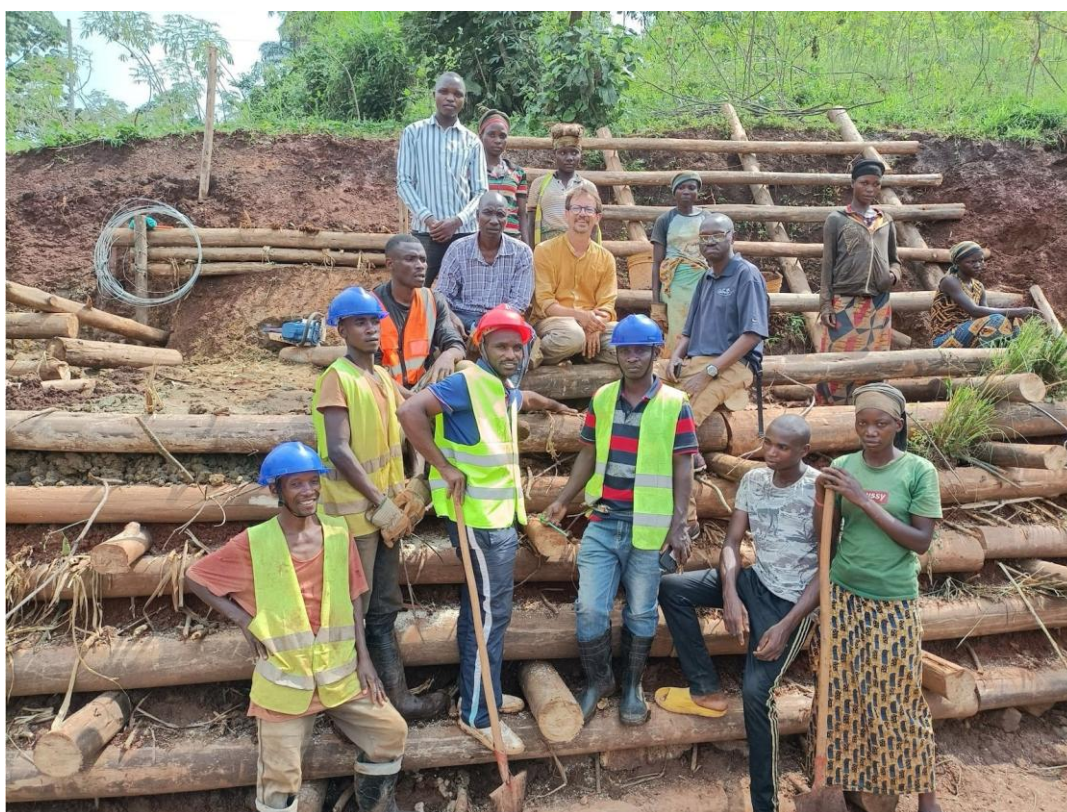
A timber crib wall built to restore land damaged by a landslide in Isare commune (Image: Preti et al, 2025, CC BY)
