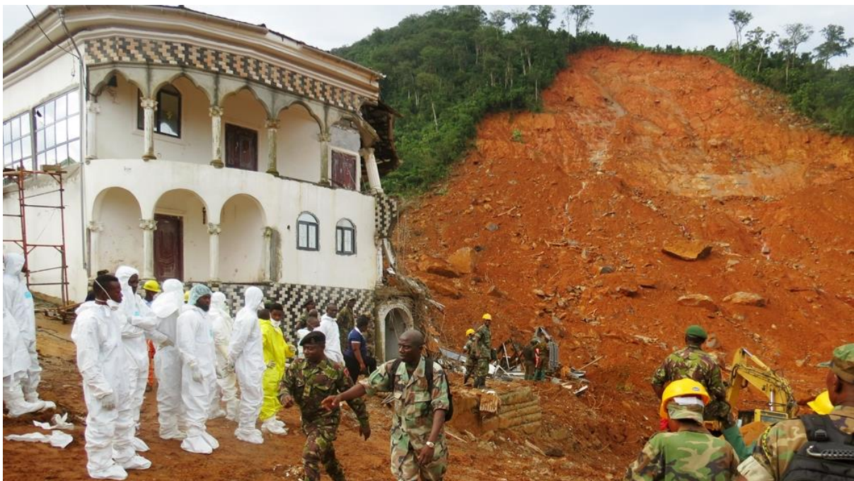
Search and rescue team members and soldiers operate near a mudslide site and damaged building near Freetown on August 15, 2017, after landslides struck the capital of the West African state, Sierra Leone [Saidu Bah/AFP]
